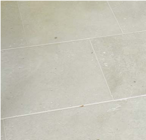
Paving 4 Porcelain Tiles - Stretcher Bond
