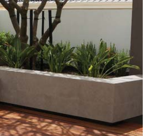
Wall Type 2 - Rendered blockwork Retaining Wall
